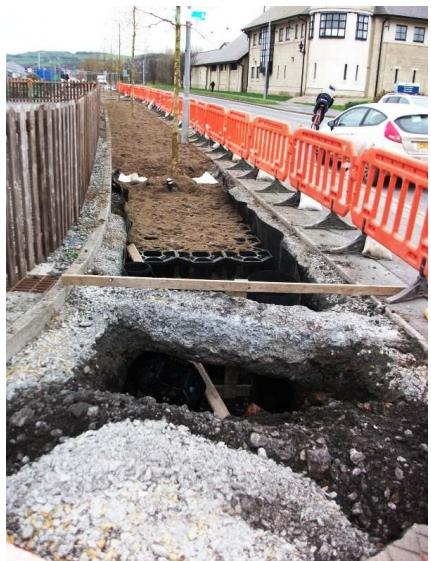
Roadside trees have been planted in Park Avenue by the Park & Ride, using a technique devised by Ceredigion's Highways, Property & Works Department. The new system combines the Stockholm Tree Planting Method, in which trees are planted in a mixture of angular rock and soil, with commercially-available plastic cell structures which can support a load of one ton per square metre. The result is a planting which fully protects trees from root compression by heavy road vehicles etc.
